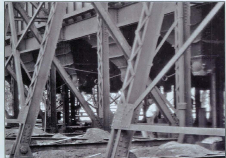
Spouts for 114 pocket hoppers in the bent-steel-supported coal storage building, each holding 70 tons of coal, are elevated 7 feet from the ground.
