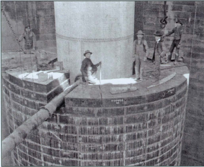
Six-ton pie-shaped cast iron segments formed a 4,200-ton ballast around the standpipe to assist holding the floor level and to prevent the building from floating during periods of high ground water.
