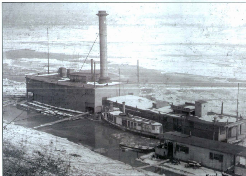
Floating a self-contained pump house seemed like a good idea to deal with a capricious river, but challenges from winter ice, summer debris, and high water caused mooring to be a significant challenge.
