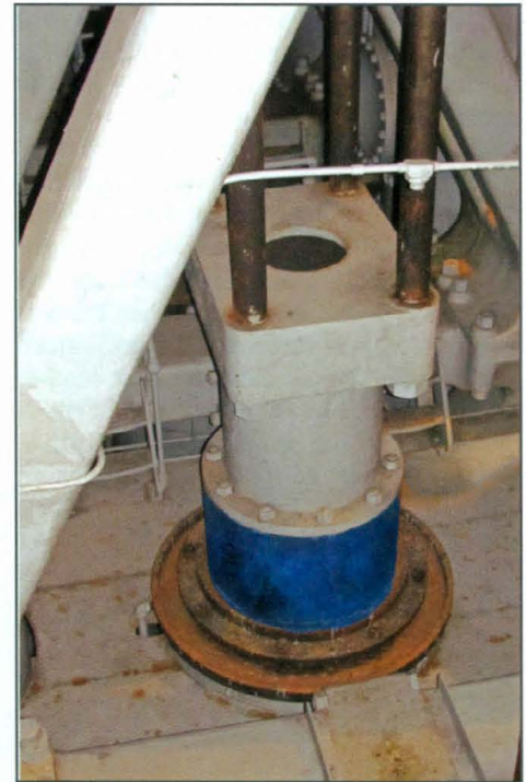
Right: The 37½-inch plunger with a 96-inch stroke is outside packed with oakum. The quad connecting rods extend to the crosshead.
