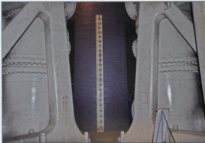
The 23-foot measuring gauge displays the water level when the pit floor is deliberately flooded at times of high ground water to prevent the building from floating.
