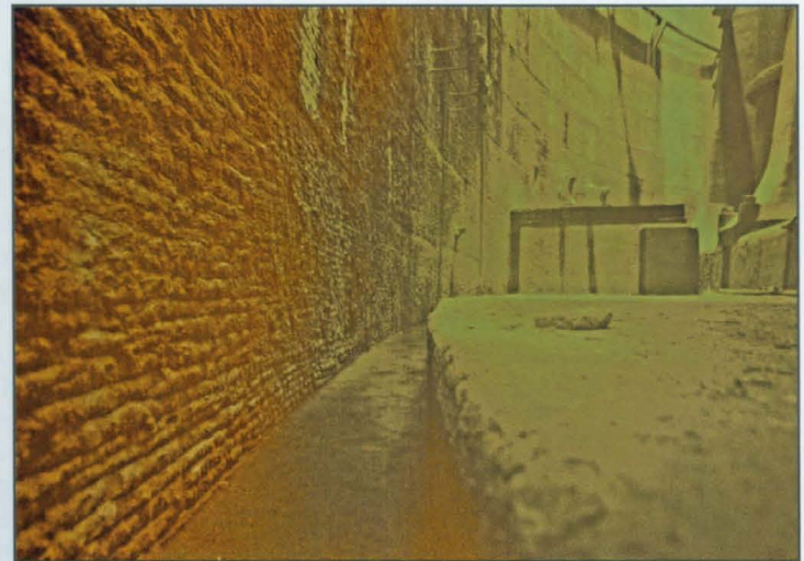
Ground water seepage was anticipated from under the 15-foot thick pit wall resting on the wooden caisson deck. This circular trough around the circumference of the pit floor captures water to be pumped outside the station.
