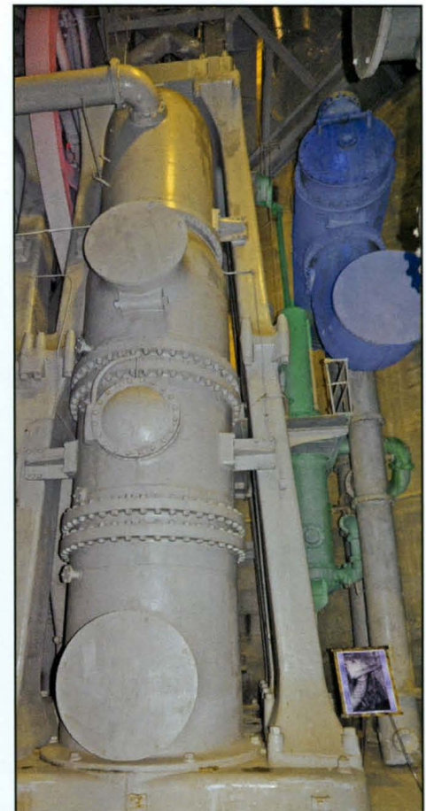
The 36-foot high pump features an inlet port, the suction and discharge poppet valve compartment, a discharge port, and a force chamber. Note the wet air pump snuggled between the surface condenser (top right) and the pump chambers.
