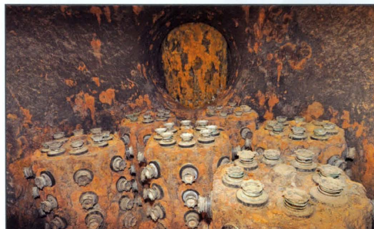
Within the suction side of the pump chamber are seven valve cages, each housing 40 poppet valves. The 37½-inch plunger, at the top of the photo, moved 450 gallons out of the station for every rotation of the flywheel.
