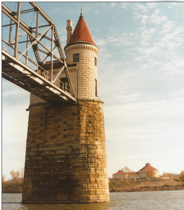
Left: The intake structure is located just off of the Kentucky bank of the Ohio River and is connected to the pumping station on the Ohio side via a 7-ft-diameter tunnel in bedrock below the river. Above: While in operation, the original raw water pumping facility required a crew of nine staff members per shift. The name plate is stamped with “1908,” but the pumps operated from October 1906 to May 1963.
