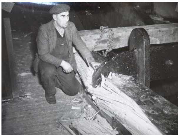
Figure 6. Smashed spring beam
