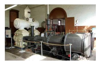
Historic Civil Engineering Landmark. Today, the entire physical plant (pumps, filters and other machinery) remain in place after more than 100 years of service and is a rare example of an intact steam water works.
