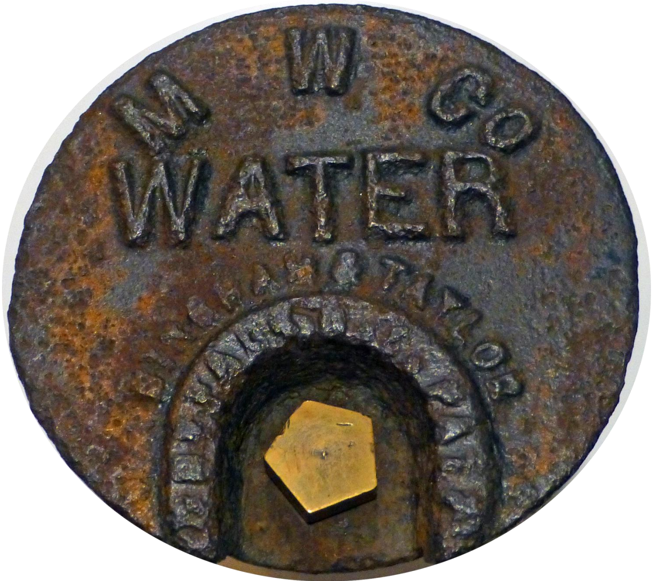
Curb box cover from the Millville Water Company
