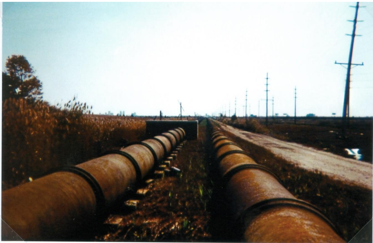
48" Cast Iron Water Mains to Atlantic City, 2002.
